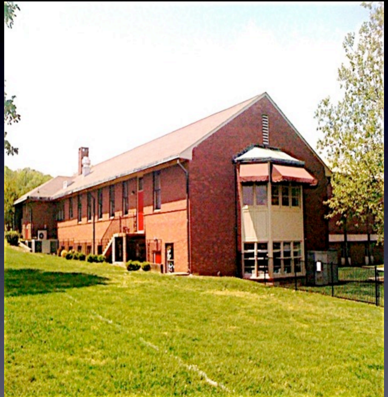
1958 First Sanctuary (now parish hall)
