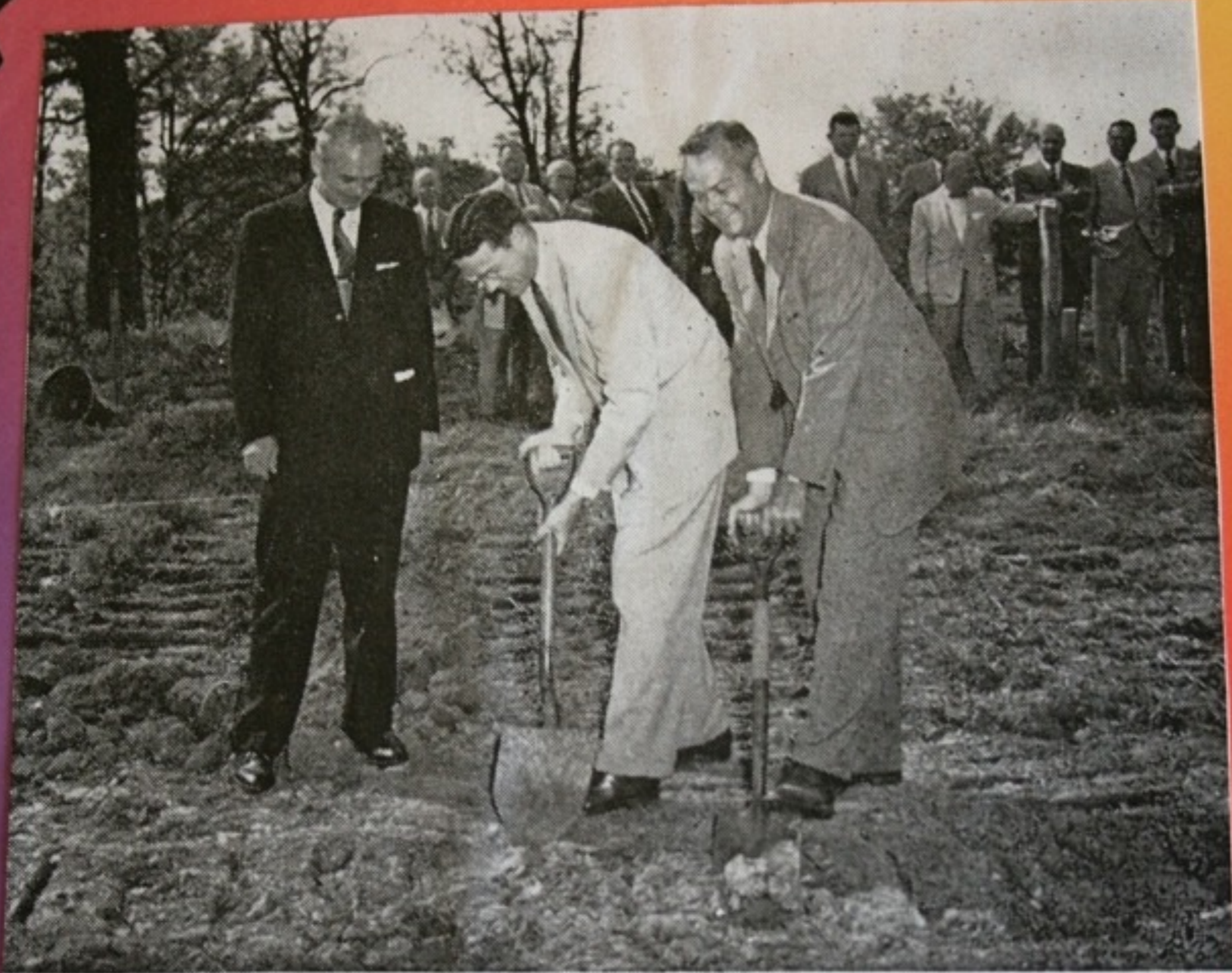
As contractor Tom Coleman and members of the Building Committee look on, Senior Warden Joseph H. Holliday, Jr., (center) and Junior Warden Louis Edge take their turn at breaking ground for the new Parish House to be built for St. Bartholomew's Church, Nashville. Ground-breaking was a part of the colorful "Beating the Bounds" ceremony held Rogation Sunday, May 6.
